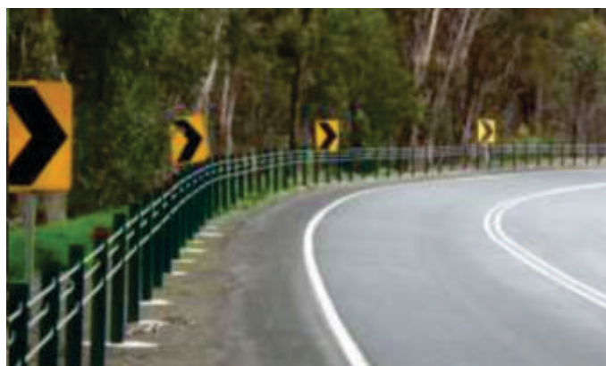
Figure 13 Plantation of shrubs along with flexi crash barrier can reduce vehicle tree collision
