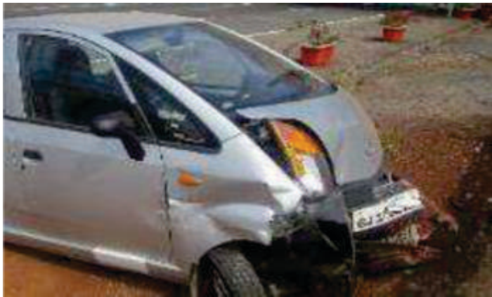
Figure 10-Impact on car due to flower pots placed in median- Mumbai Pune Expressway
