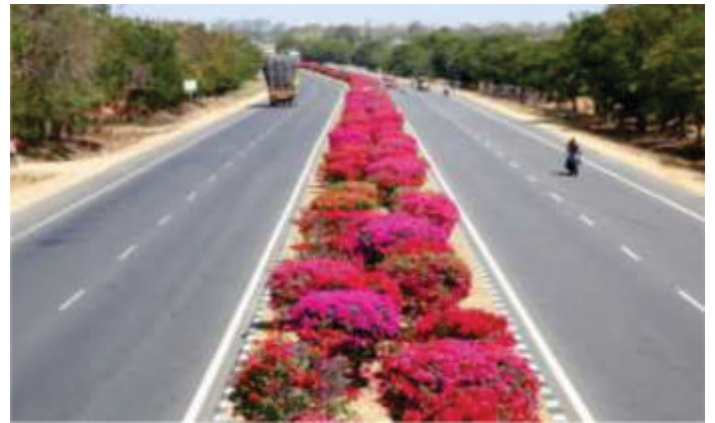
Figure 11-Shrubs can be planted instead of pots in medians of to act as cushion & Ant glare-NH 44, Nagpur Hyderabad Expressway
