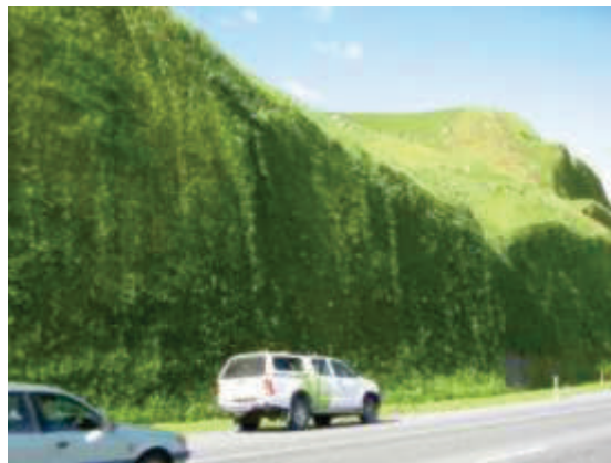
Figure 20. Hydro seeding used for slope stabilization
