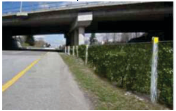
Figure 6 Plantation of shrubs along with flexi wire crash barrier can be explored (indicative)
