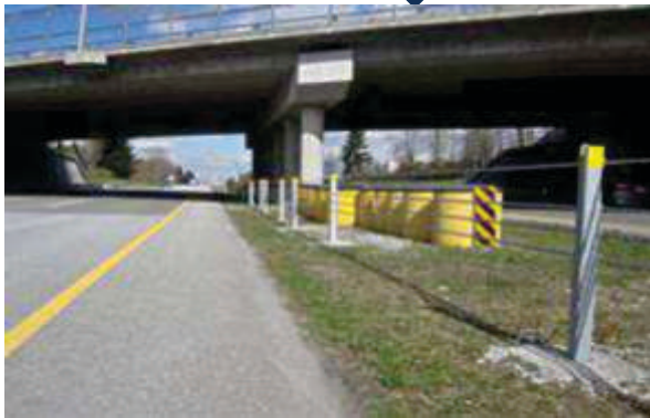
Figure 5 Space required for crash attenuators (IRC: SP: 84-2014)
